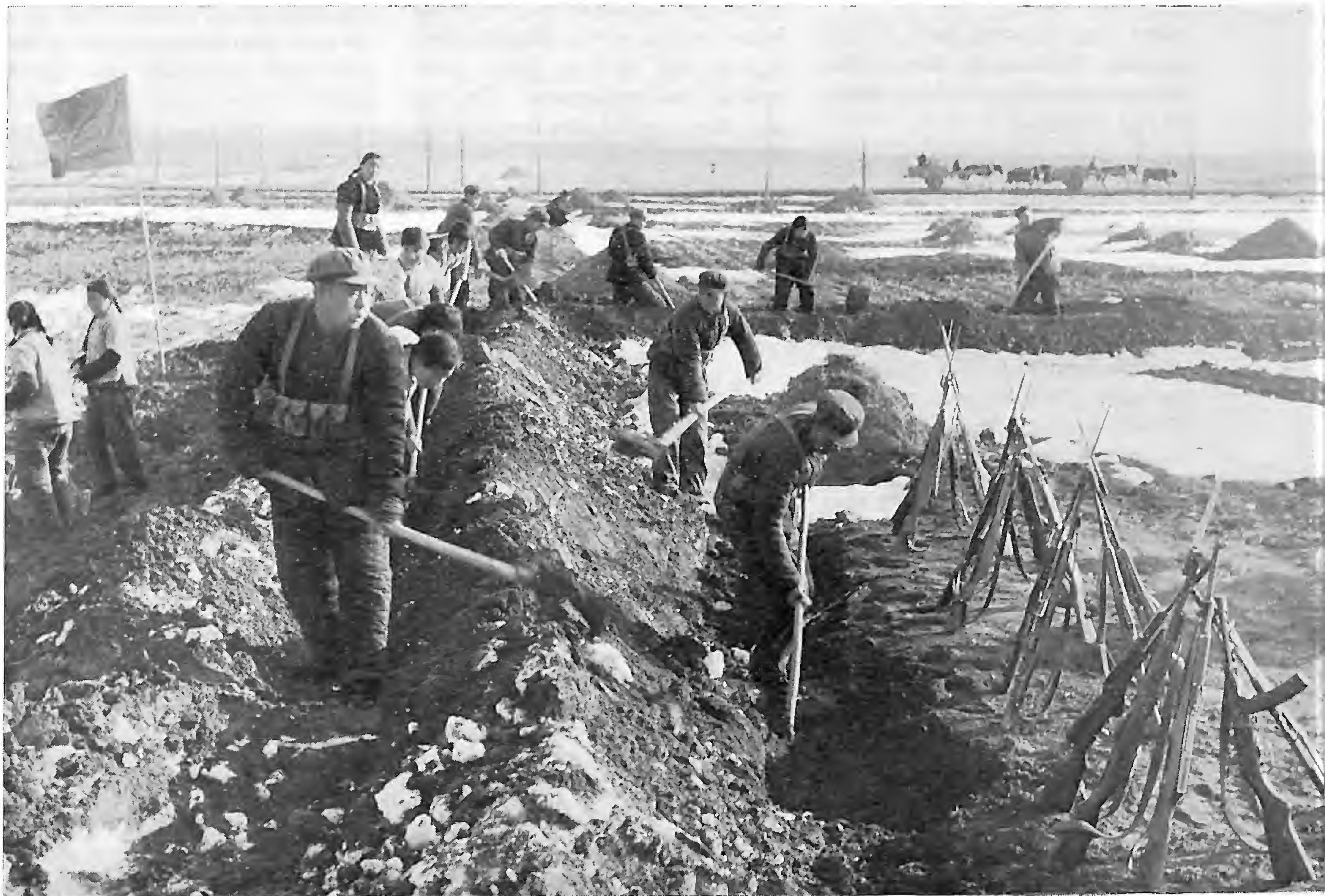
Hao Huai-yu (left) leads in work and drill.
